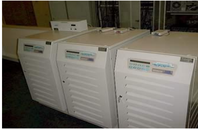
شكل (5-11) جهاز UPS True On Line Double Conversion
